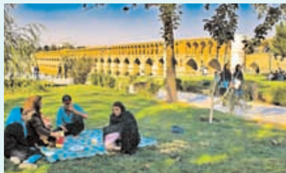
Isfahan, Ponte Khaju
